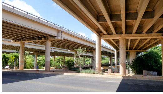
Figure 3.13: Frame structure. Roberta Crenshaw Bridge, Austin, TX.
