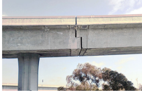
Figure 3.5: Gerber Beam. Near the interchange of I110 and I105, Los Angeles, CA, USA.
