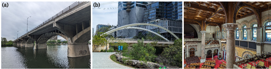
Figure 3.17: Arch structures. (a) South Congress Bridge, Austin, TX. (b) Butterfly Bridge, Austin, TX. (c) The Assembly Chamber at New York State Capitol, Albany, NY.
